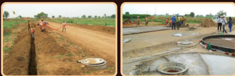
Actual Site Images Construction in full swing at Hyde Park Estate
